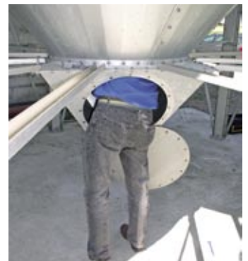
Auger box with manhole
