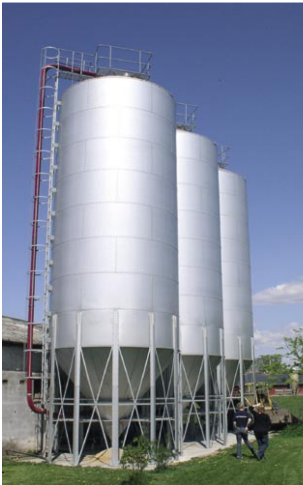
Unique XB-silo equipped for dry storage with air inflow pipe and cyclone.
