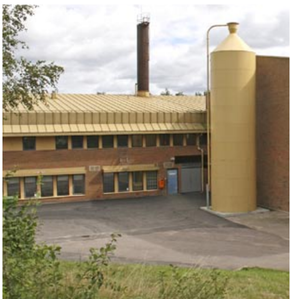
Painted MAFA BIB 67 silo (66.9 m 3 ), at Veinge school.
