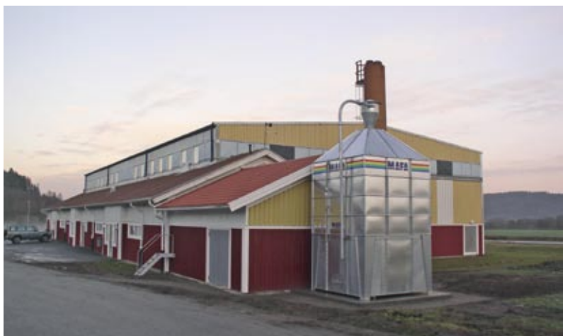
MAFA outdoor module silo (28.9 m 3 ) at Strömsholm school.
